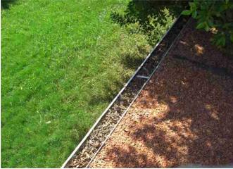
The gutters need to be serviced, such as resealing them, sealing seams, etc.
